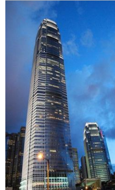
Location: Hong Kong Owner: Sun Hung Kai Prop. & Henderson Land
